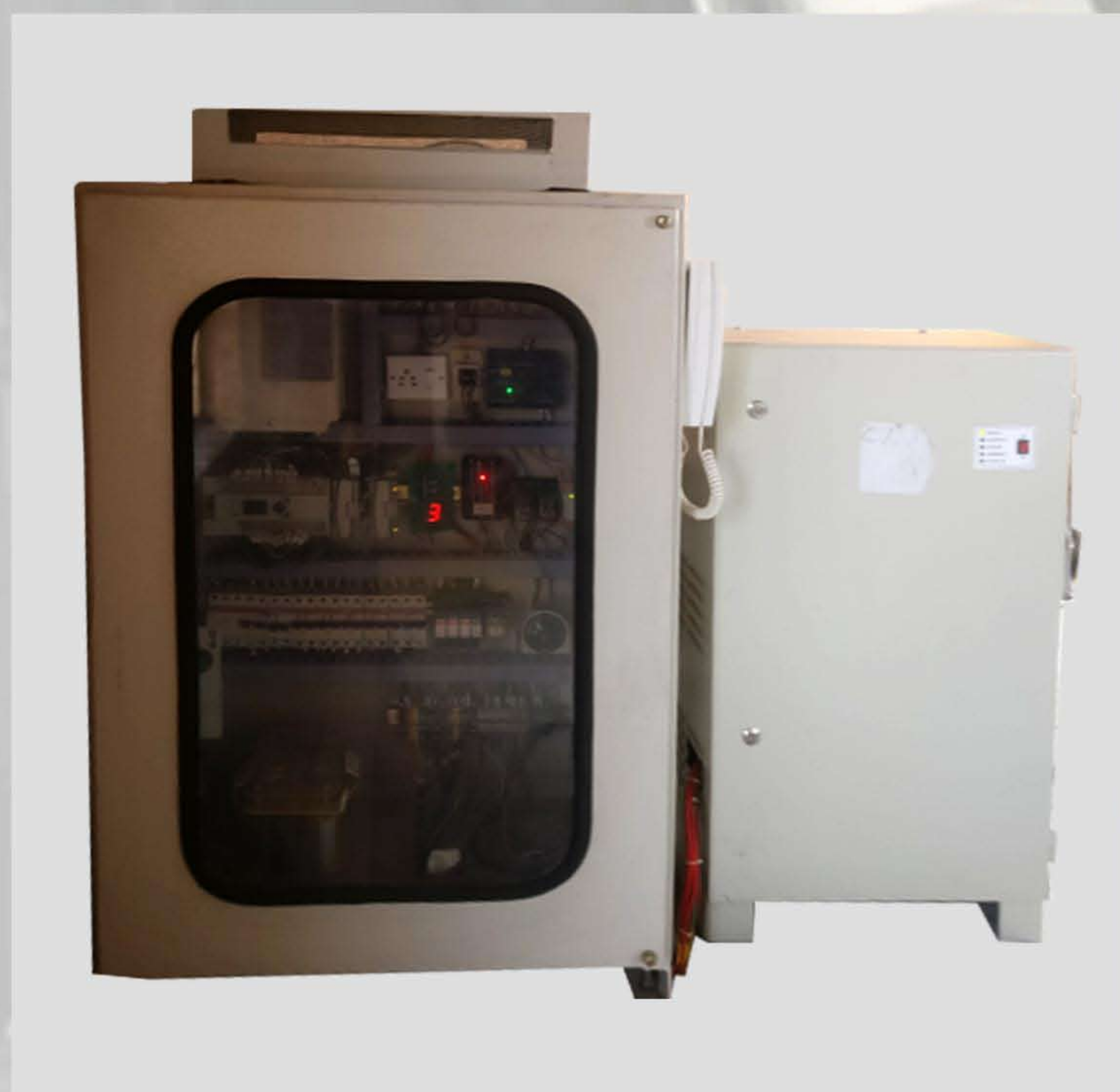
PLC And ARD Panel In Operation
